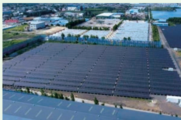
Distributed photovoltaic panel in Xinglongzhuang Coal Mine
